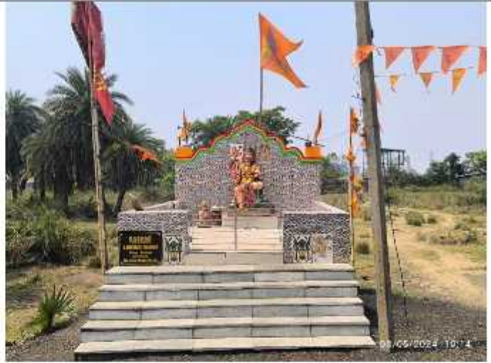
Construction of Hanuman Temple at Kantapal
